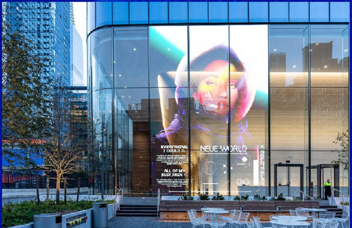
(Picture of glass curtain wall of the building)
